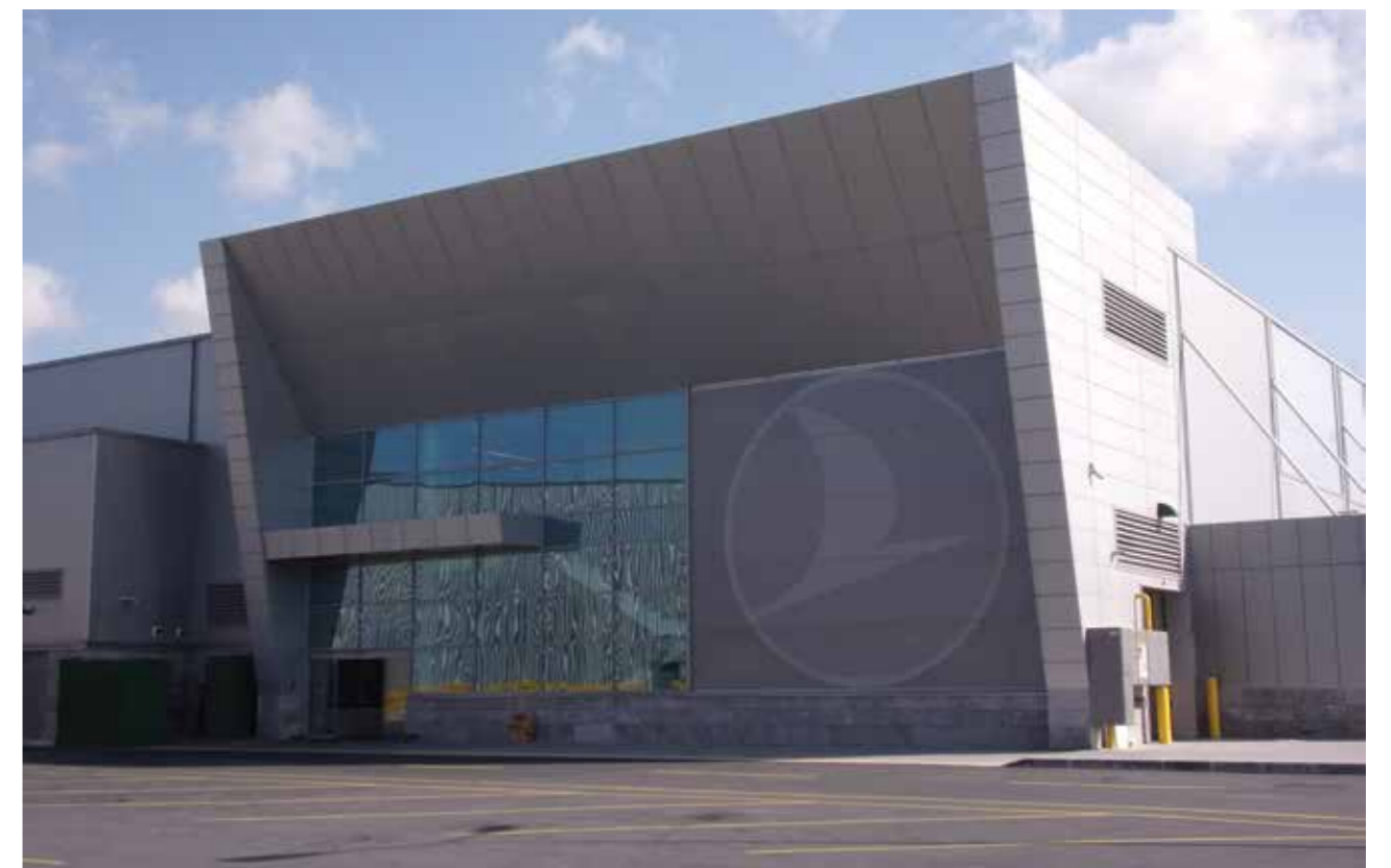
Perforated THY logo on painted aluminium sheets are designed as sun shading element on the entrance façade in compliance with glass glazing, aluminium composite panels and ceiling.
