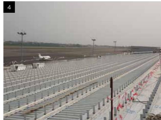
4. The halter clips are installed on the top hats. It is very critical for the standing seam installation, the halters should be in correct place.
